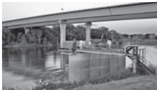
George Kristoff Water Treatment Plant Sacramento River Intake Pumps
