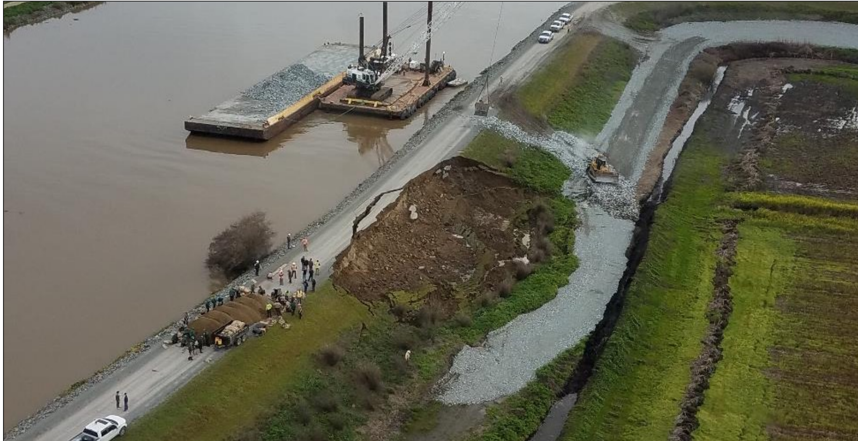
Levee Repair
